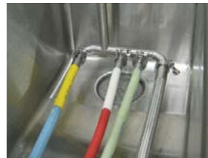
Clean interior and exterior of hoses
